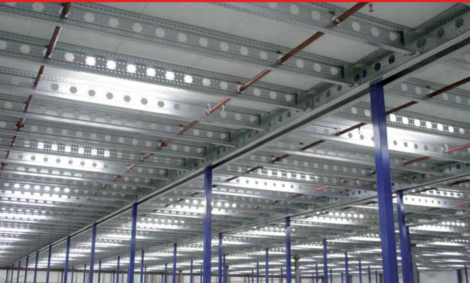
Unique Nolte Mezzanine floor profile hexagonal hole pattern for sprinkler pipe installation.
